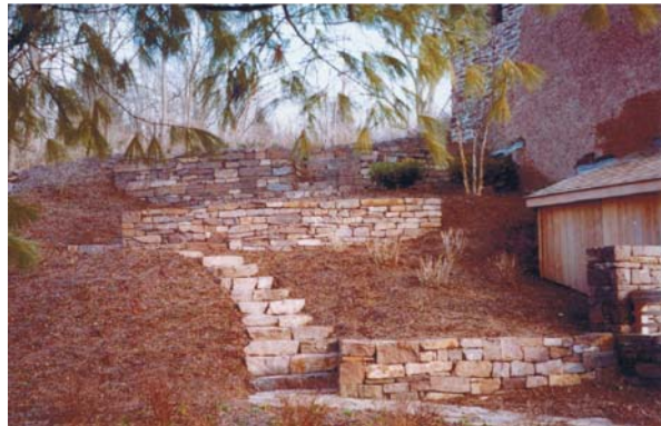
After shot of hillside near barn with terraced walls and pathway.
